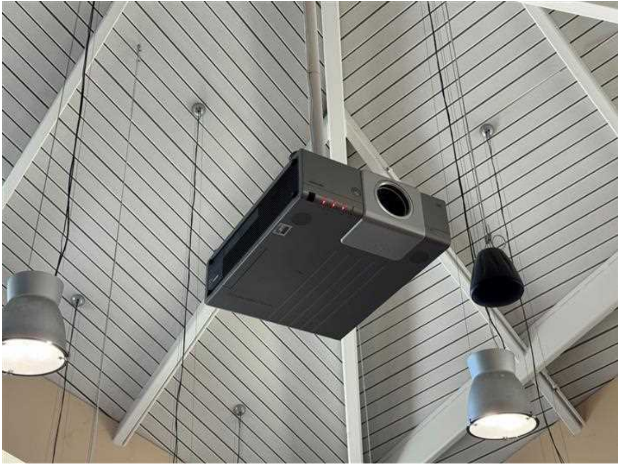
Overhead projector. The project bulbs are no longer available, and it can no longer be controlled. The black cone shaped speaker is also visible. There are six speakers hanging from the ceiling in the room.
