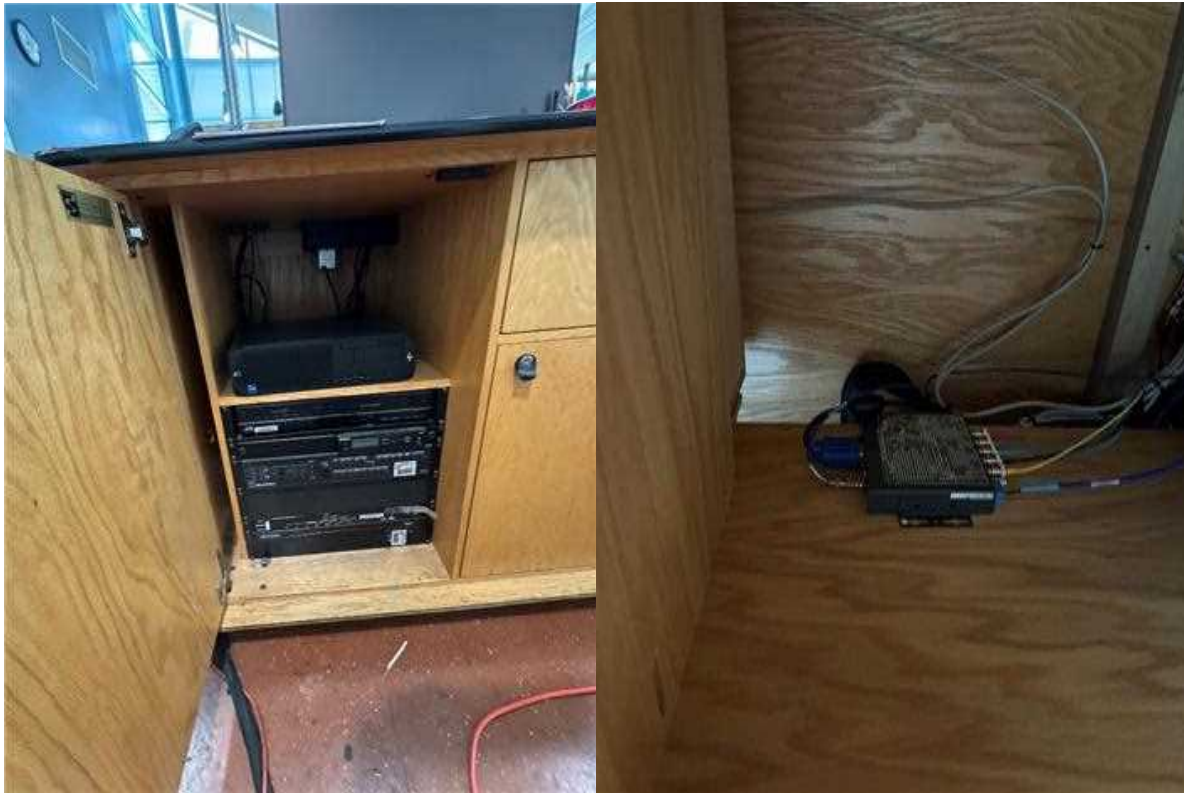
(Left) Equipment inside the podium for switching between various A/V sources. (Right) RCA cables that connect the projector to the podium. These cables will have to be replaced with updated HDMI cables.
