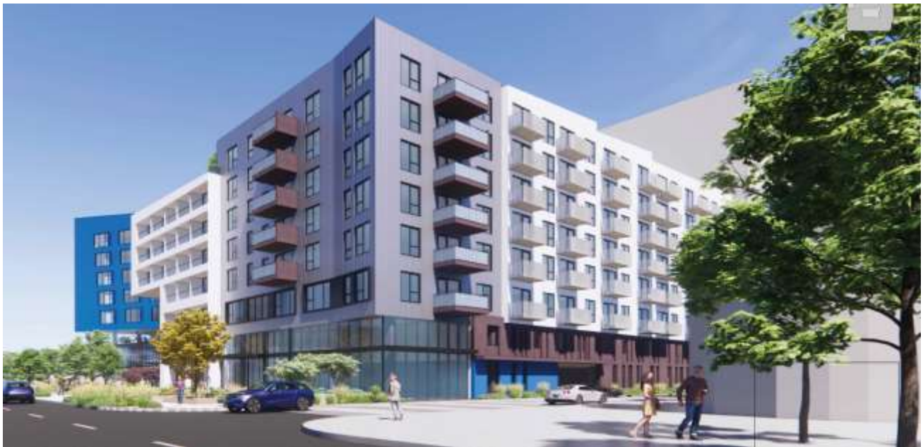
The south façade (to the right) will also have three “sections” to visually break up the bulk of the structure, as well as a white saw-tooth roofline over the middle section of the building to eliminate the visual monotony of a straight roofline, and an angled edge that relates to the “sheared” wing frontage (in blue) at the corner of Victory and Canoga.
