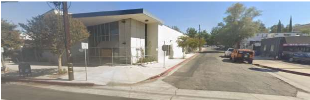
View of the existing vacant bank structure at the corner of Ventura Blvd. and Rigoletto Street.
