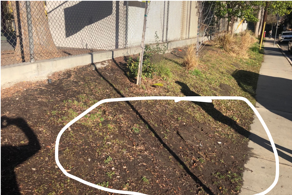
Notice bare dirt and dirt seepage onto walkways
