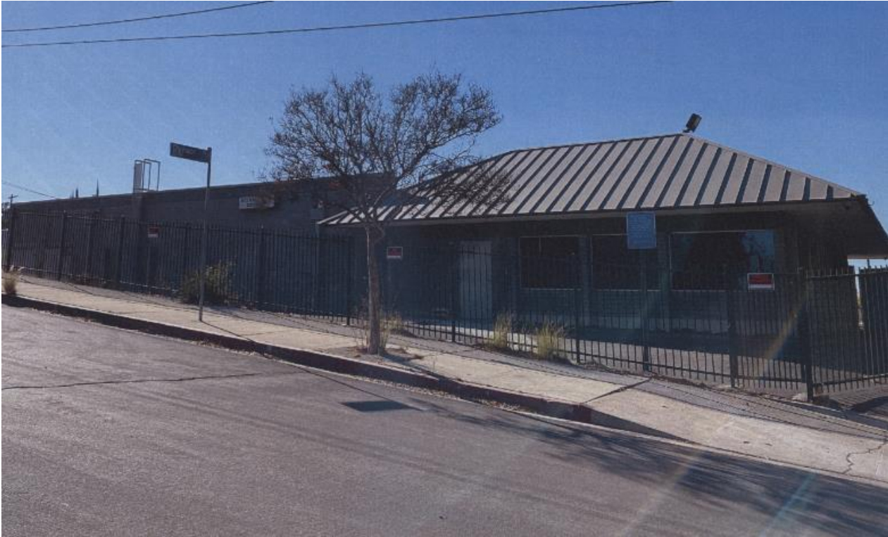
5425 Farralone Avenue (existing)
