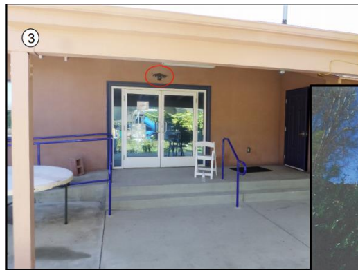
③ Exterior mounted wall light shielded from neighboring residential.
