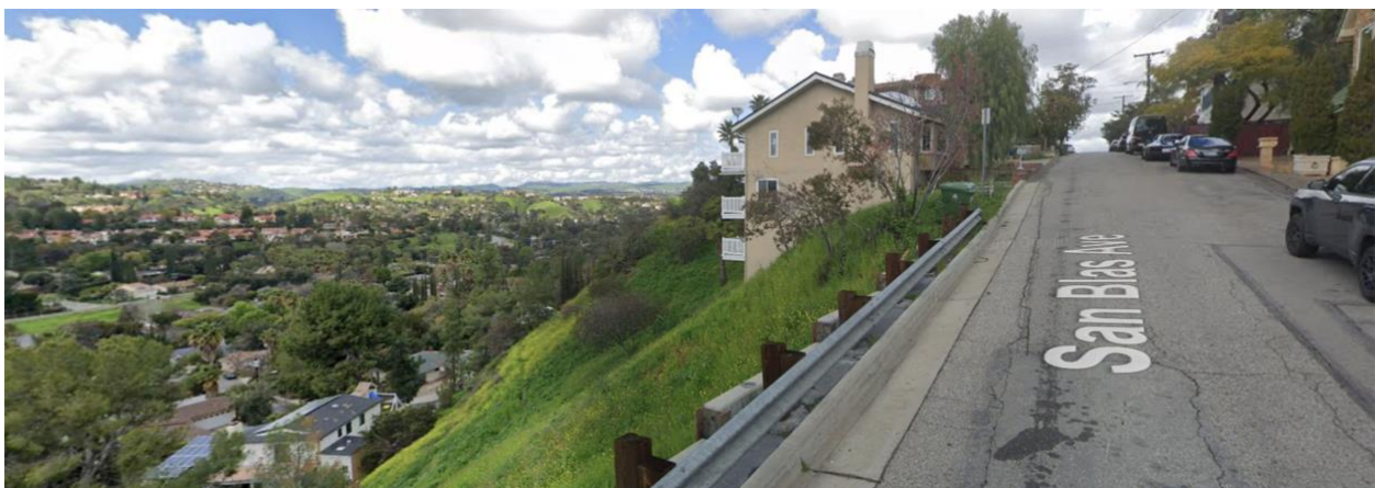
Street view of site which is at center of photo
