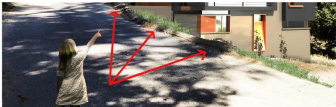
Natural berm along roadway to channel water away from site and prevent slides
