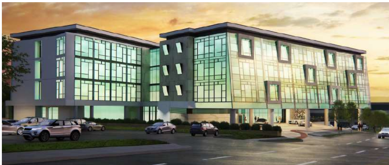
West and east facades from Ventura Blvd. showing motor court area, mosaic window treatment and “frames” for windows.
