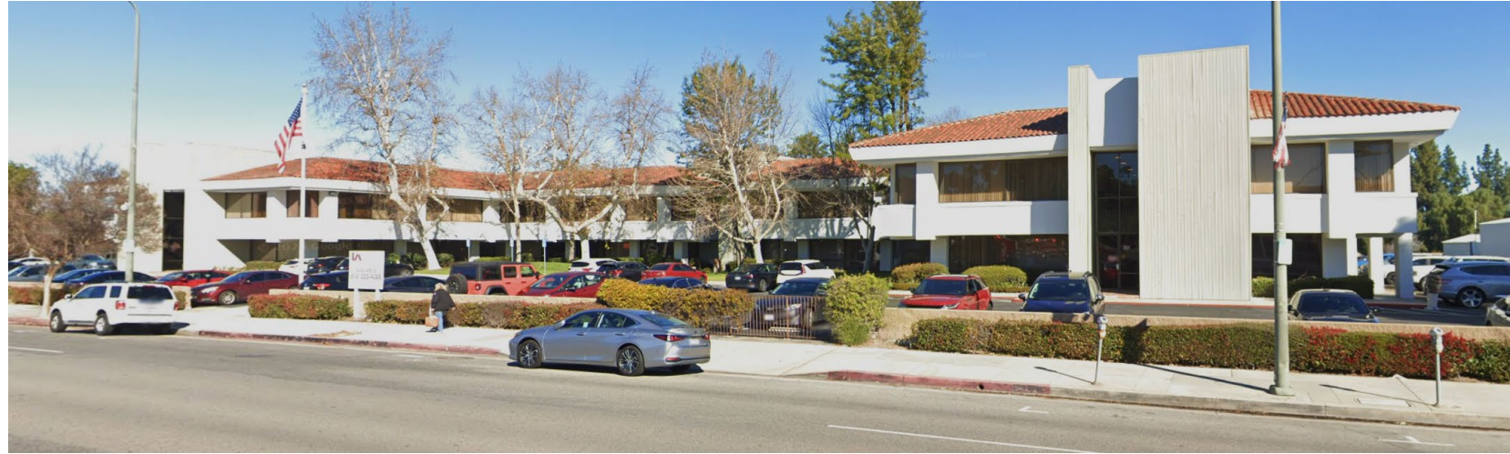
Project Site / Existing Building (21241 Ventura Boulevard)
