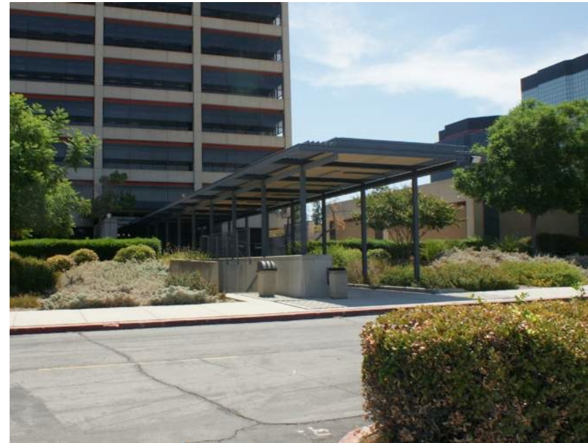
5. OFFICE TOWER WEST ENTRANCE CANOPY
