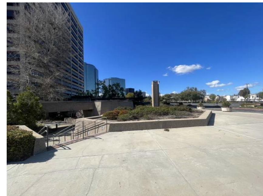
9. ENTRY STAIR TO OFFICE BASEMENT
