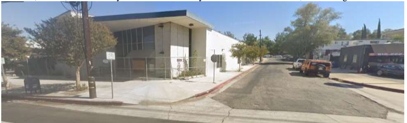
View of the existing vacant bank structure at the corner of Ventura Blvd. and Rigoletto Street.
