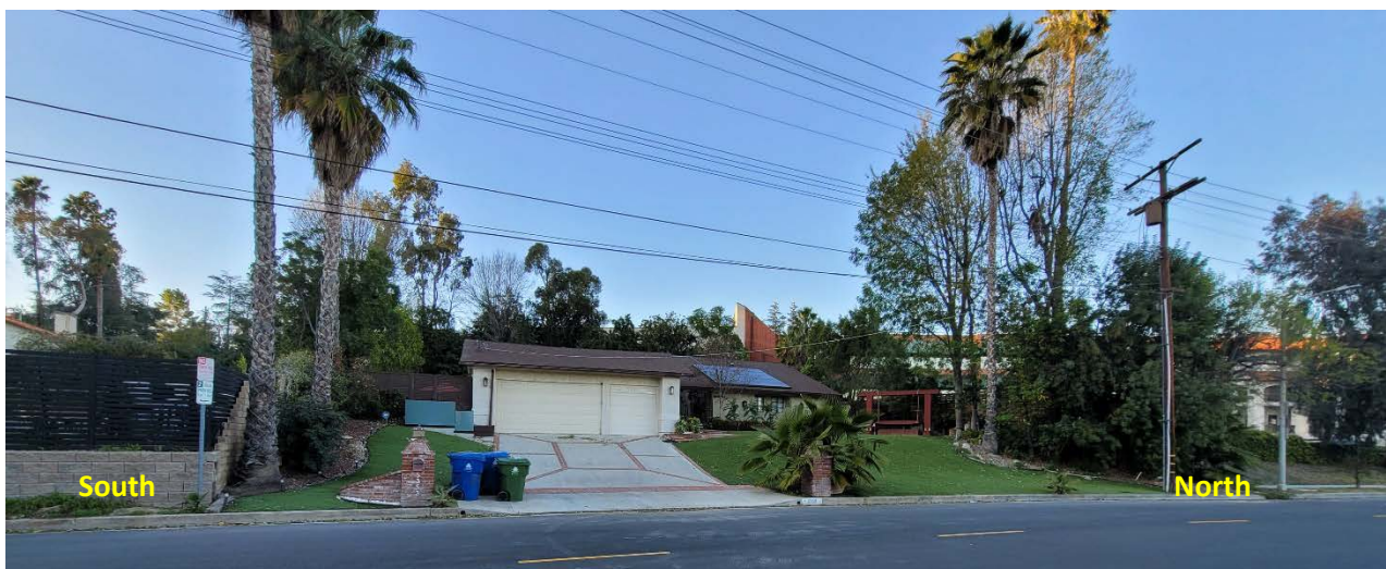
View of the existing SFR on Del Moreno Dr.
