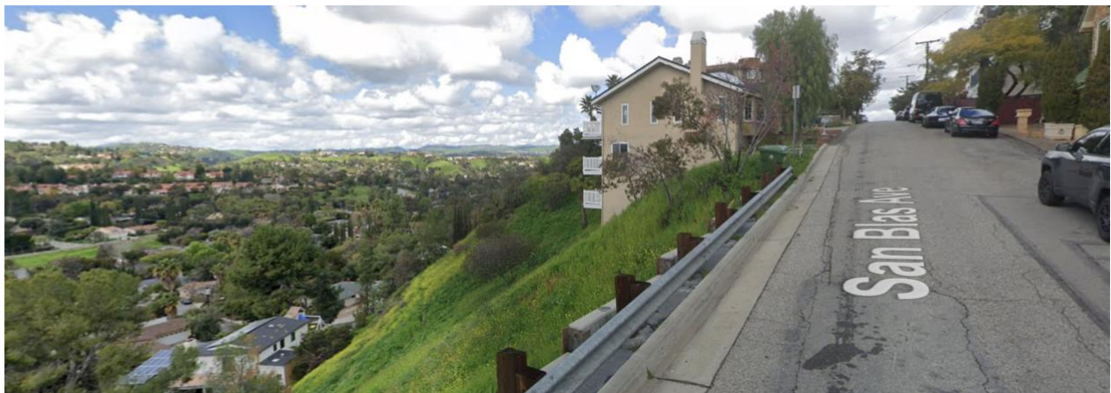
Street view of site at center of photo
