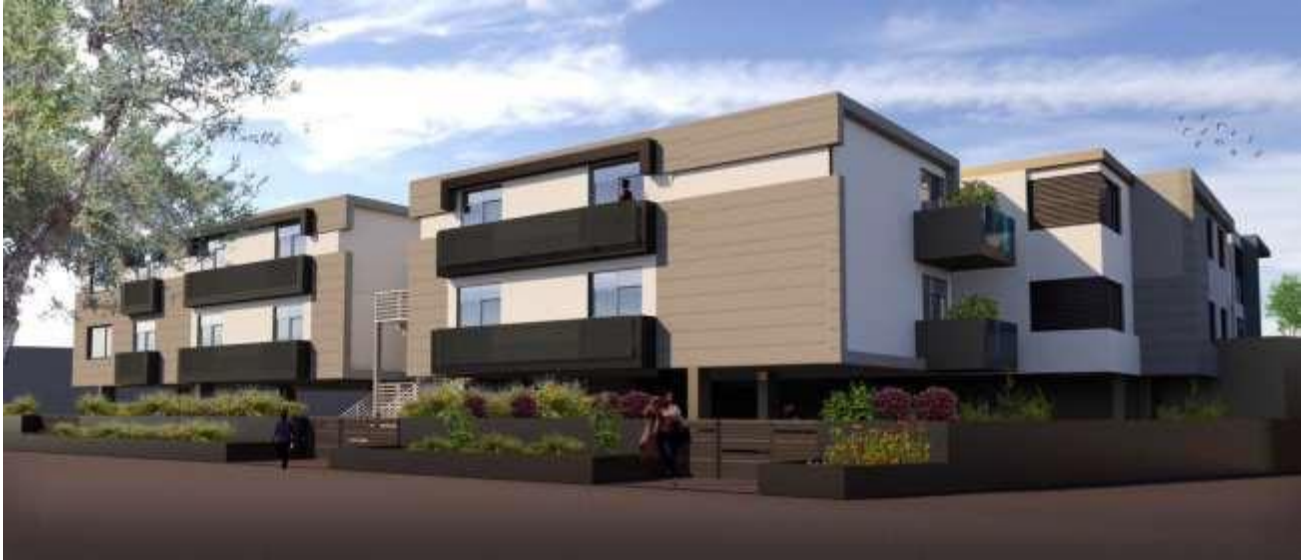
North (rear) facade facing 101 Freeway.
